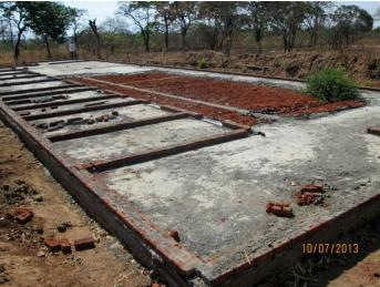
The full foundation and floor slab were installed by the middle of 2013. Walls and roof were then completed.
